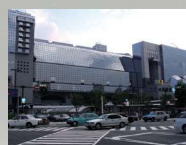
K station building
