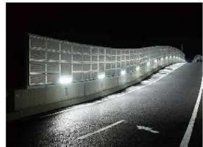
防護網ブロック [目地材 (止水性)] Safety wall blocks [joint materials (water-sealing)]
