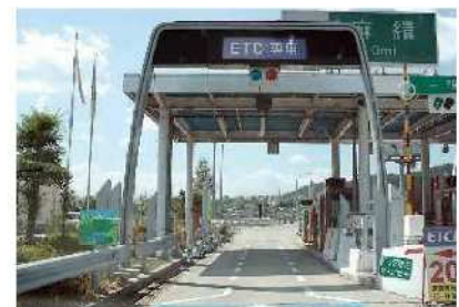
ETCゲート [電波吸収体 (導電性ポリエチレンフォーム)] ETC gate [radio wave absorber (conductive polyethylene foam)]
